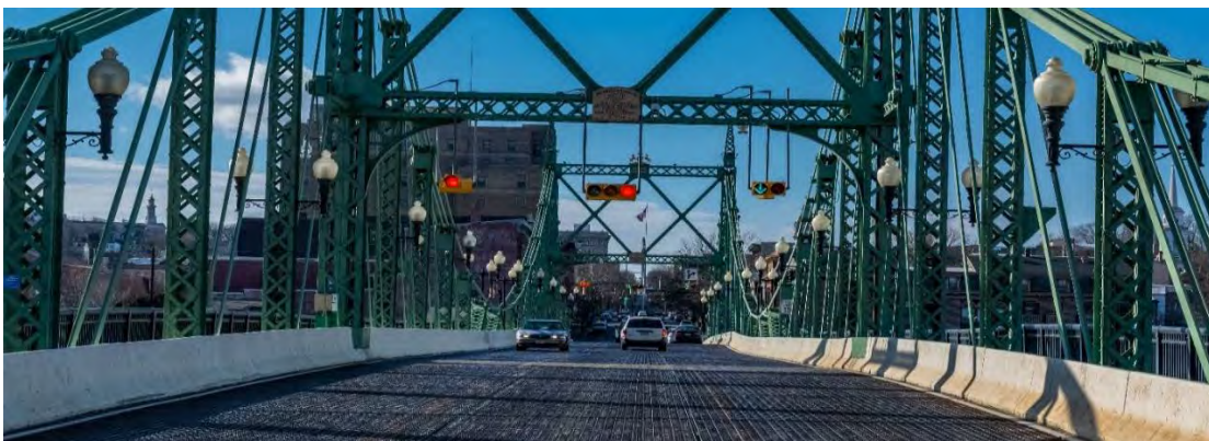
Northampton Street Bridge (3-ton limit), Phillipsburg
