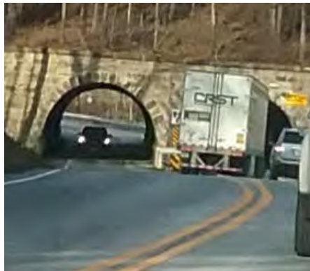
Truck Stuck in CR 519 Tunnel
