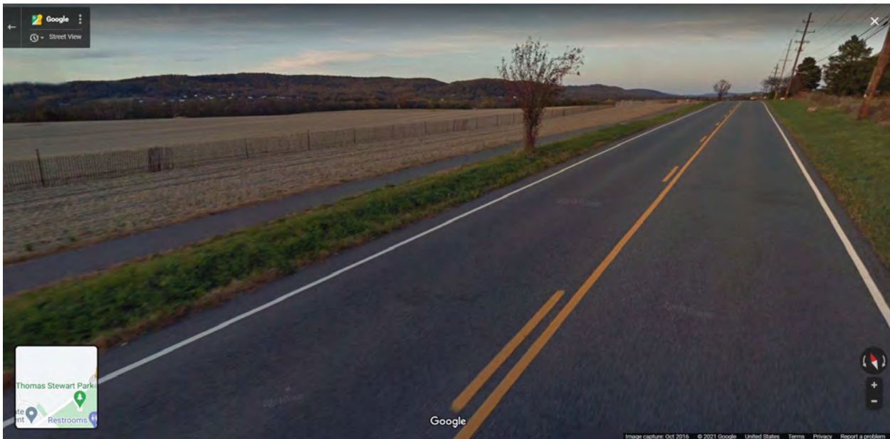
CR 638 Sidepath, Greenwich Township
