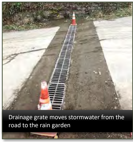
Preparing for rain garden installation
